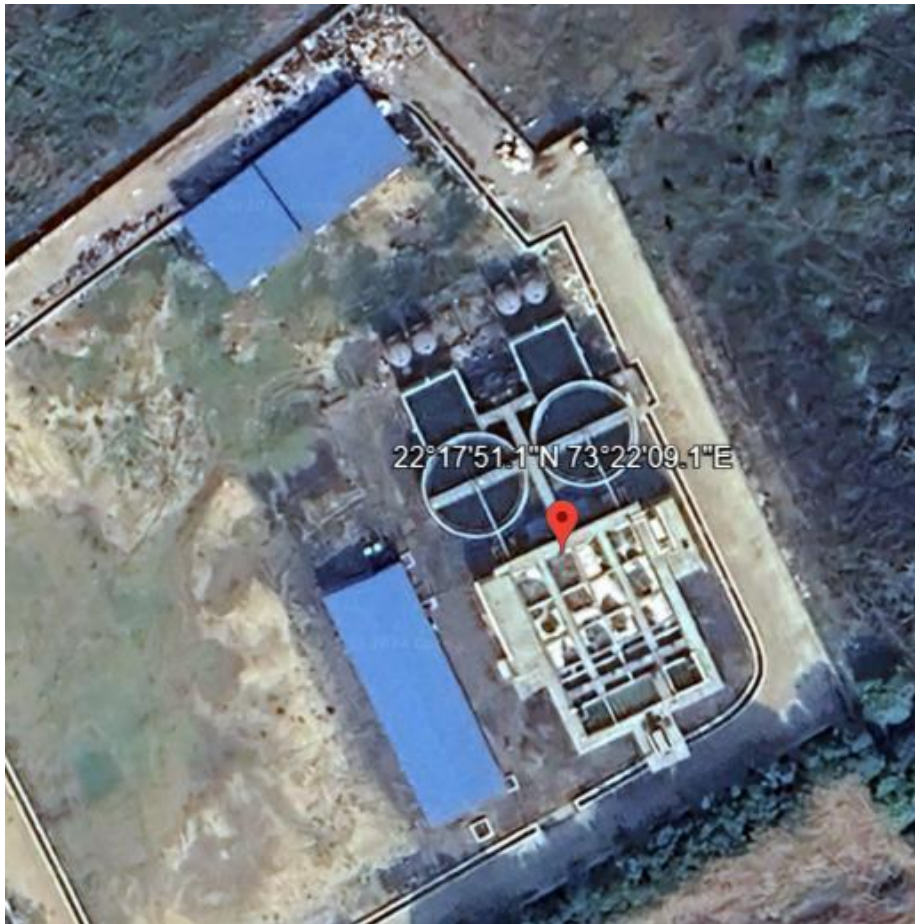
* STP Wastewater Recycling by Parul University
